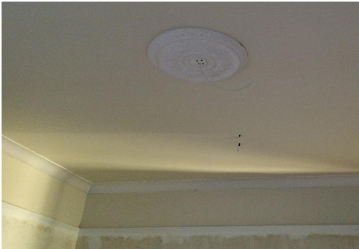
Figure 9: Areas of completed clay paint
