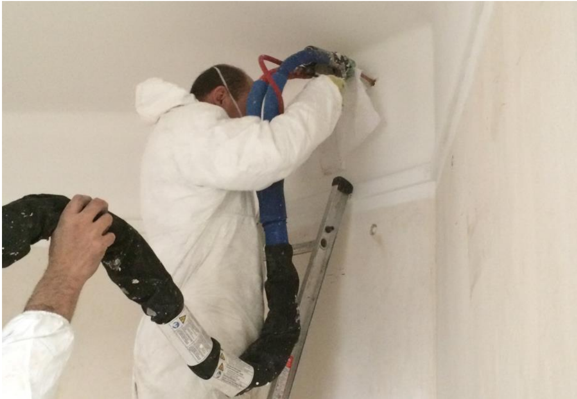
Figure 5: Installing the foam insulation
