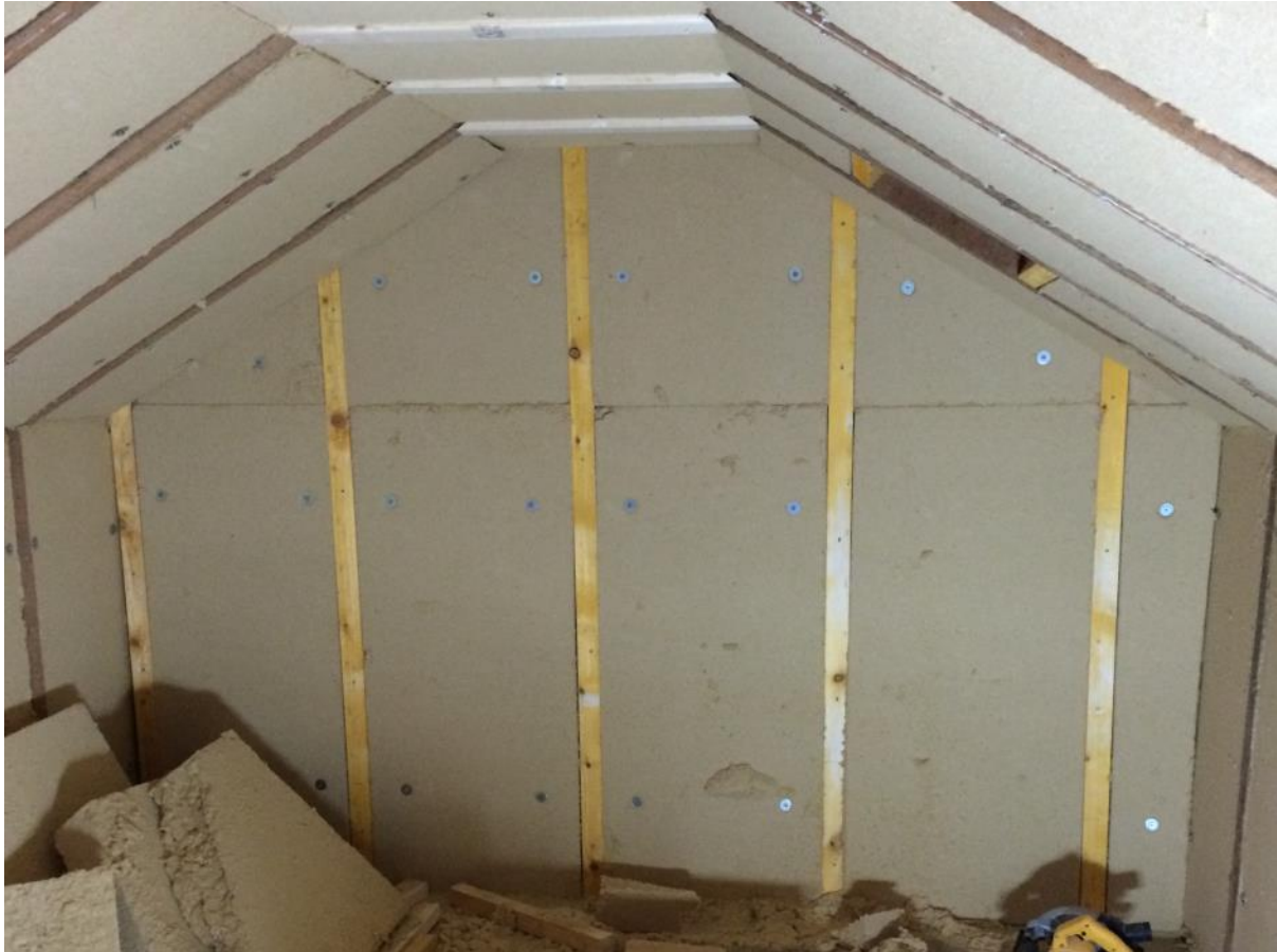
Figure 7: The wood fibre insulation installed in the roof space
