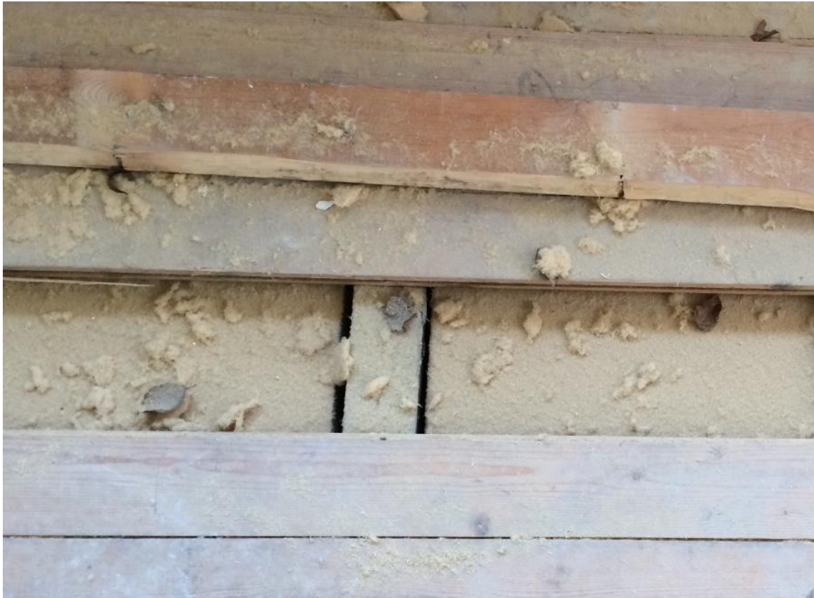
Figure 6: Wood fibre board insulation installed between the floor joists.
